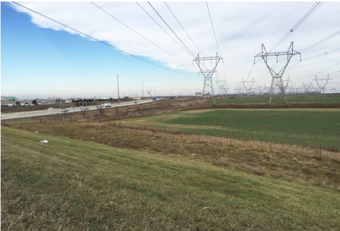
Photograph #14: Looking east from Torbram Road along the proposed runningway route, where it will pass between 407 ETR and the hydro transmission corridor.
